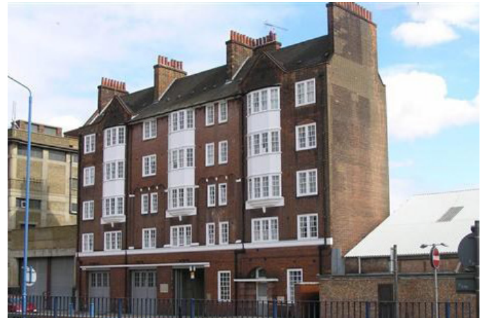
The Acme Fire Station © Acme Archive
